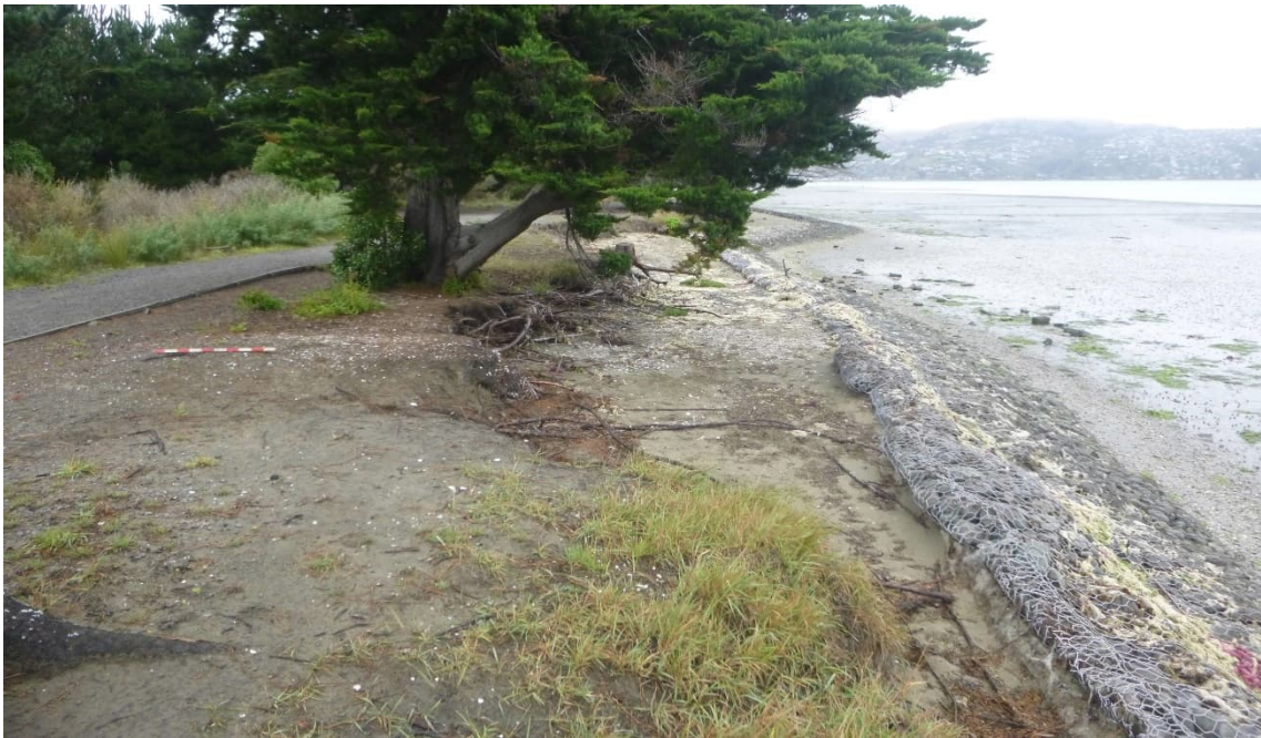
Figure 7-17. Looking south along the estuary shoreline showing the path (far left), exposed midden (scale stick shows approximate location of surface material), eroded bank (mid ground), and reno mattress (far right). Scale is in 100 mm increments.
