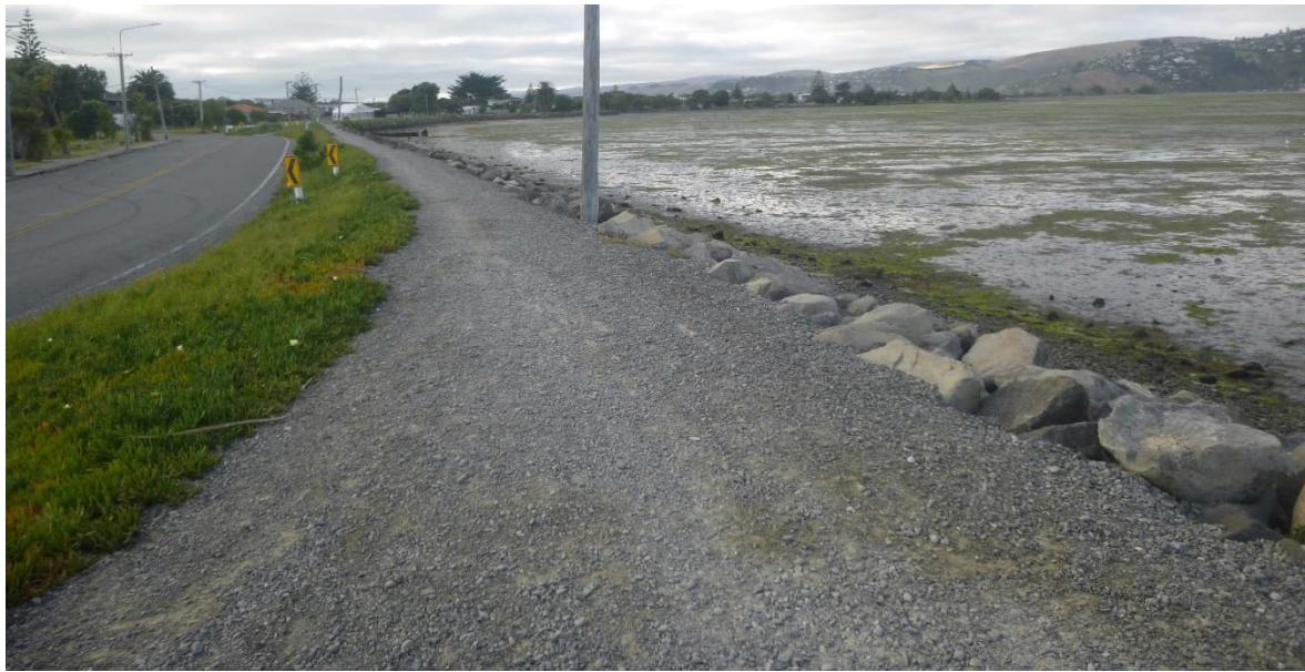
Figure 7-42. Facing south, showing walkway along Ebbtide Street. The estuary is on the right.
