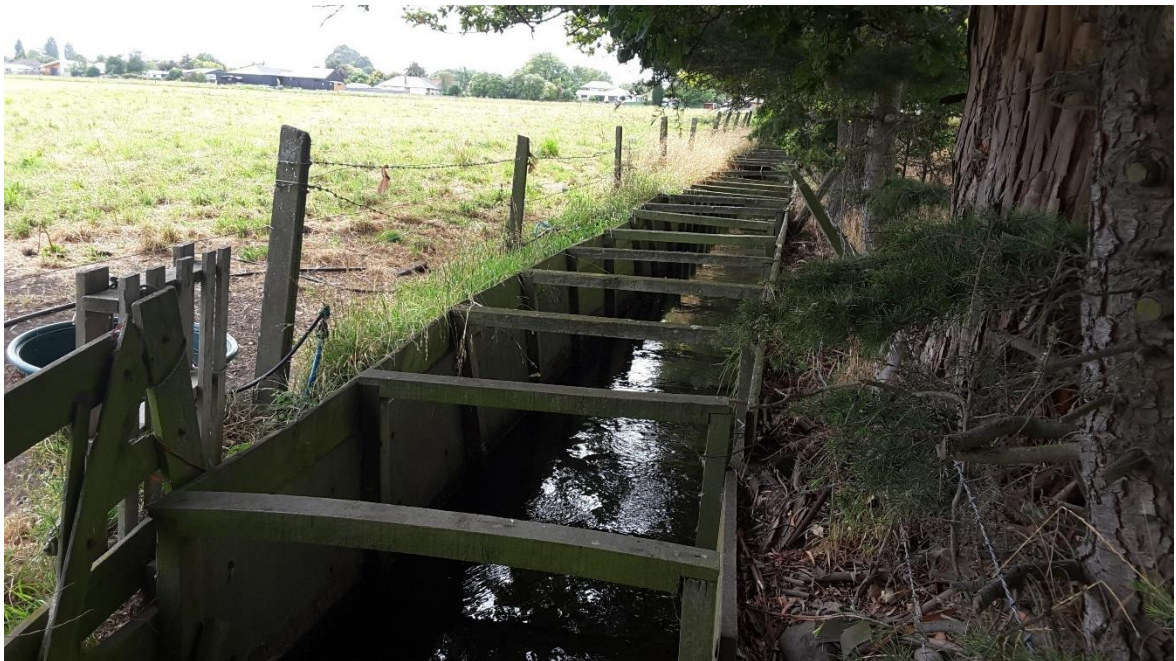
D) Box drain at the northern boundary of 240 Cashmere Road
