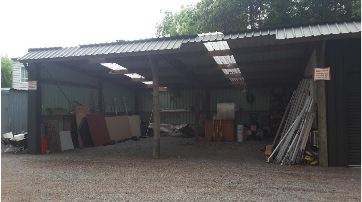
I) Pole shed at 236A Cashmere Road
