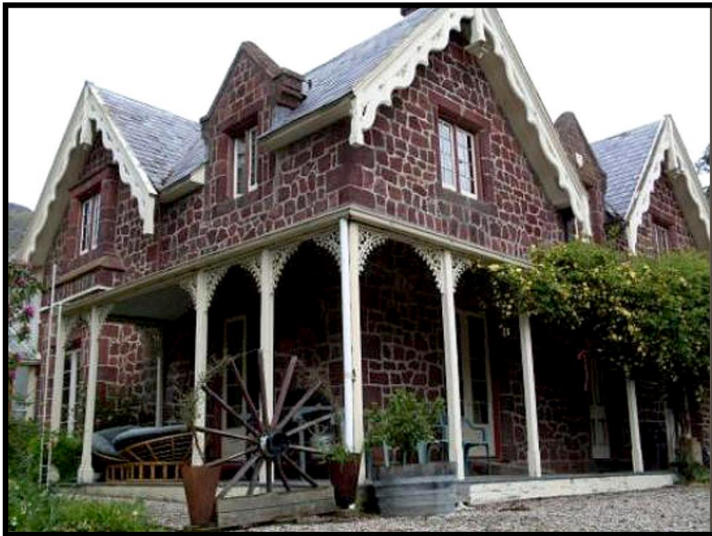
The Pūrau Homestead. Source: Heritage NZ
