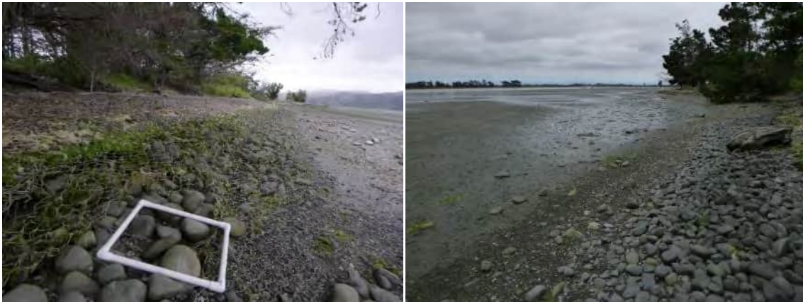
Figure 8. Cobble material (either loose or retained by reno mattresses) along the estuary edge and on the adjacent seabed at South New Brighton Park.
