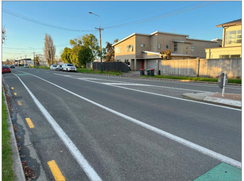
Photograph 6: Madras Street north of Purchas Street
