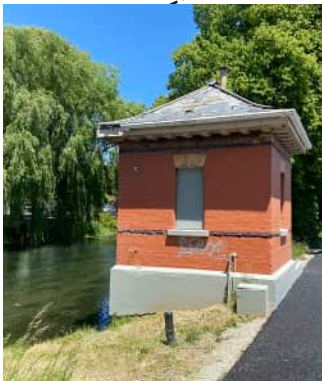
Historic pump station.
