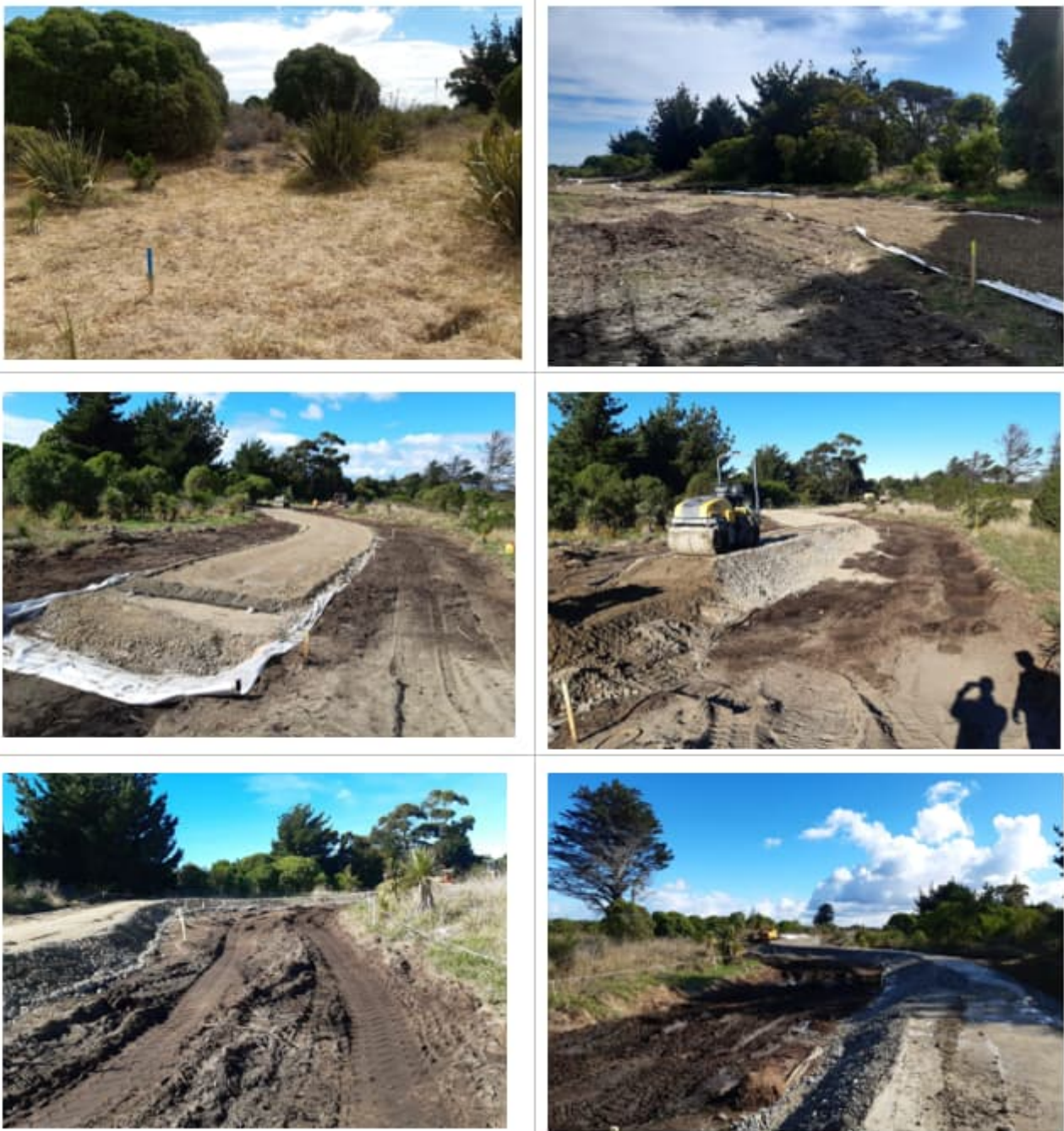
Figure 44 Example photographs of stages of construction of the Bridge Street inundation bund, which is similar to the proposed Southshore/SNBP bund (source Citycare)
