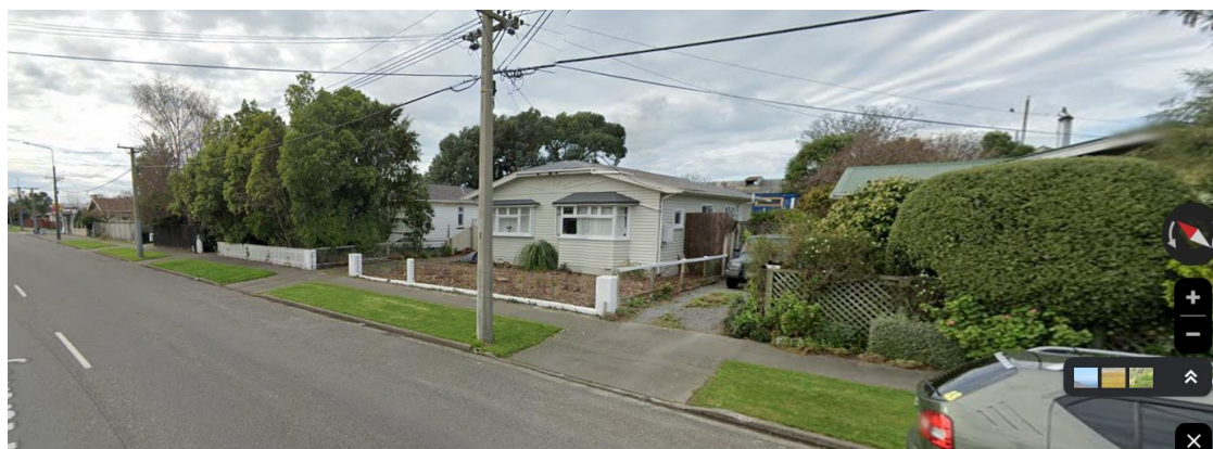
Figure 1: East side of Radley St (121, 119, 117 Radley St) – Zoned 'Industrial General'
