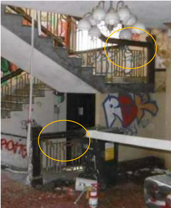
Short sections of balustrade on lower landings
