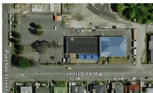
Figure 11: Aerial photo of adjacent Korean Presbyterian Church.
