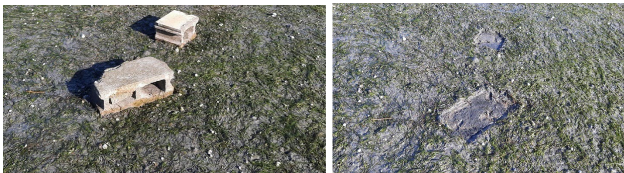
Figure 2. Seagrass smothered by debris released from derelict erosion protection structures along the estuary edge.
