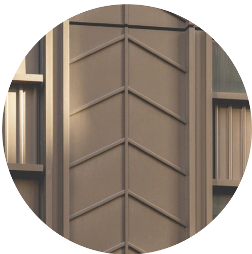
M1 BRONZE METAL CLADDING & DETAIL
