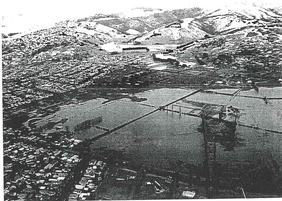
411 Hendersons Road ponding area (Southeast)
