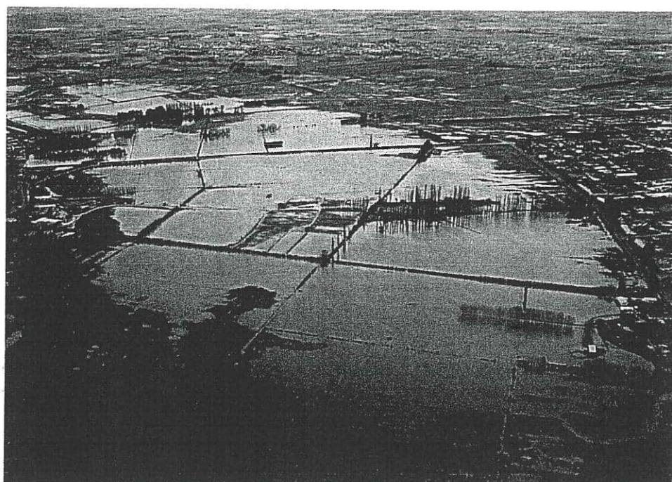
408 Hendersons Road ponding area (Southwest)
