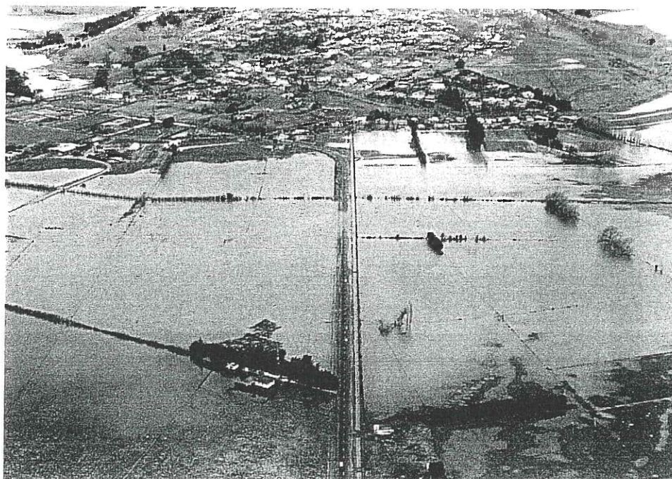
412 Hendersons Road ponding area (Southeast)
