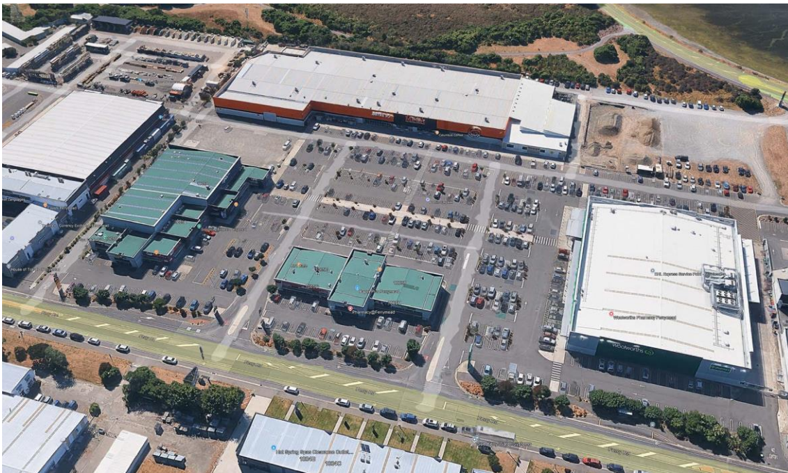
Figure 1 Woolworths Ferrymead (building at right) seen associated with two separate groups of shops (green rooves). While the expansive carpark is partly concealed by buildings, the supermarket does not have good street appeal (rotated perpendicular to Ferry Road) and the various buildings are still 'islands' to a degree, surrounded by hardstand and bisected by internal traffic lanes. Pedestrian connectivity from Ferry Road is also very poor. Note lack of any public park space.
