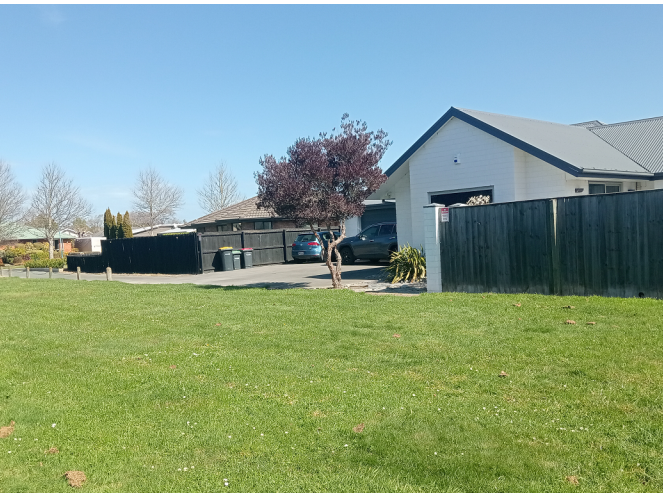
VIEW #2 - Transition from tall fence to no fence to post and cable. Ake ake on boundary. Providing passive surveillance to the reserve
