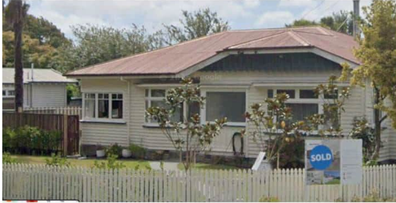
Figure 9: Site's original house's facade facing Gosset Street
