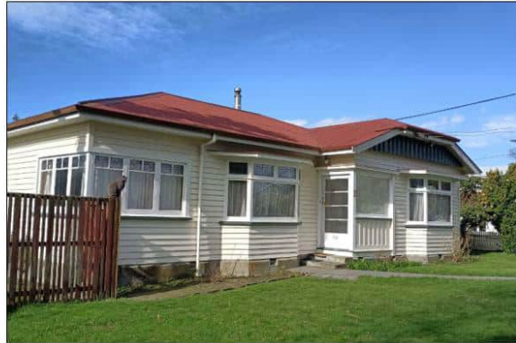
Figure 7. Western and part of the northern façade of the dwelling.
