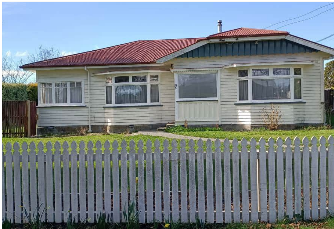
The western façade of the dwelling from the road boundary looking east. Taken by the planner during the site visit.
