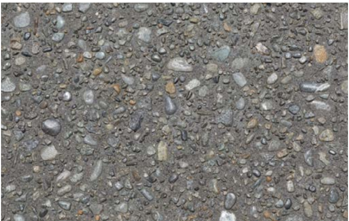
Exposed aggregate concrete / feature paving / vehicle threshold paving
