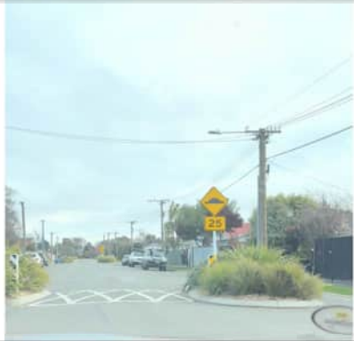
Passageway narrowed. Series of raised and painted road areas. Low speed limit. Multiple warning signs.
