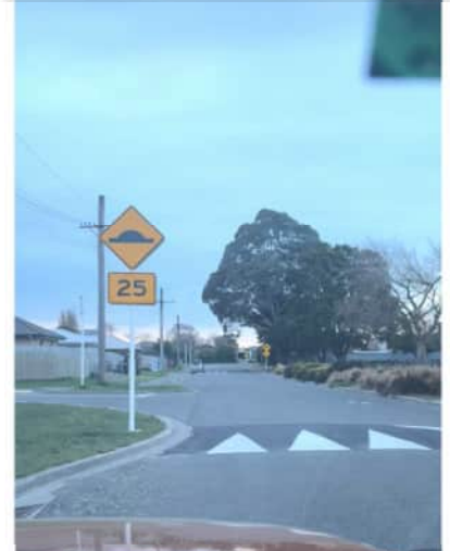
Passageway narrowed. Series of painted speed humps. Low speed limit. Multiple warning signs.
