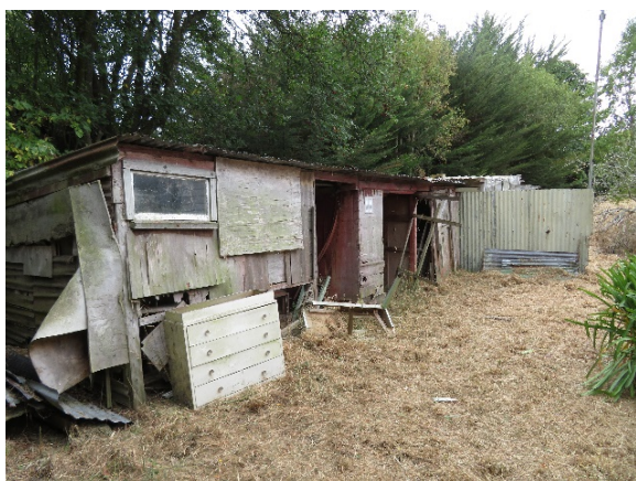
Figure 138: Source: T Ussher 01.2020 The sheds to the north side of the house.
