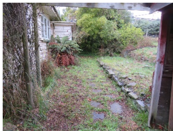
Figure 139: Source: T Ussher 06.2021 The stone paving and terrace edging to the south side of the house.
