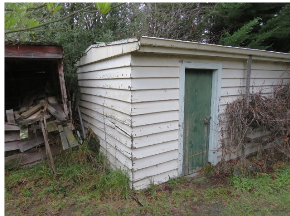
Figure 137: Source: T Ussher 06.2021 The garage and woodshed.
