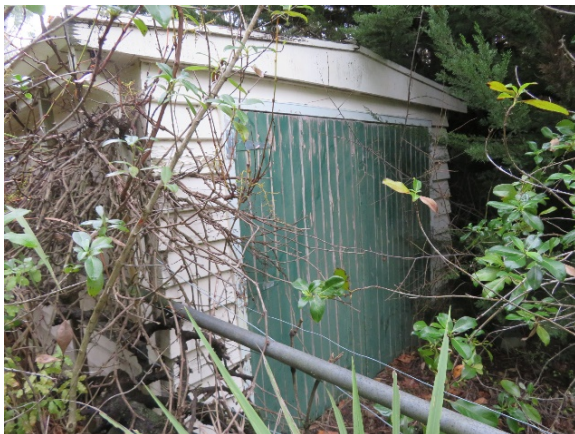
Figure 136: Source: T Ussher 06.2021 The street frontage of the garage.
