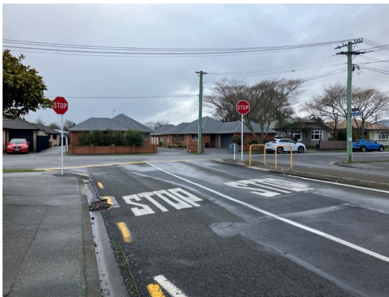
Photo view of the Athelstan Street / Simeon Street intersection (Athelstan Street approach)
