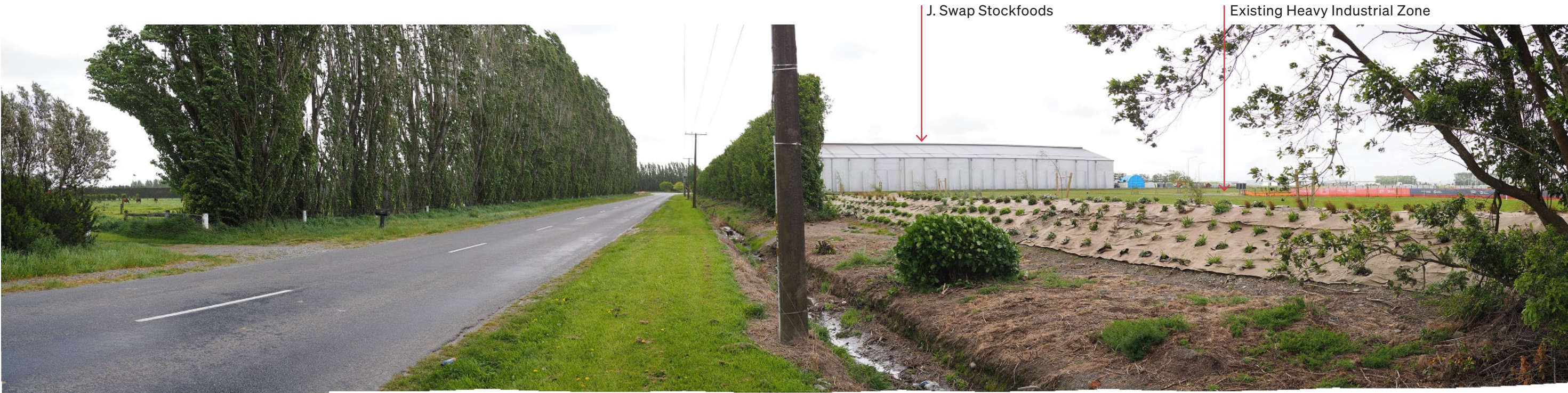
Viewpoint 8: Located along Marshs Road, east of the J. Swap Stockfoods property. The juvanile plants on the earthmound are in accordance within the ODP, which is proposed within the site, which is 960m away.
