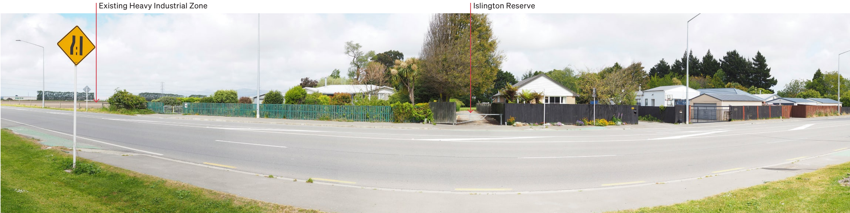
Viewpoint5: Located beside the Alpine View Holiday Park along Main South Road, looking south towards the existing Heavy Industrial Zone, the entrance to the Islington Reserve, and the residential properties within the site. The PPC will allow for industrial development to replace these dwellings, which is 75m away.
