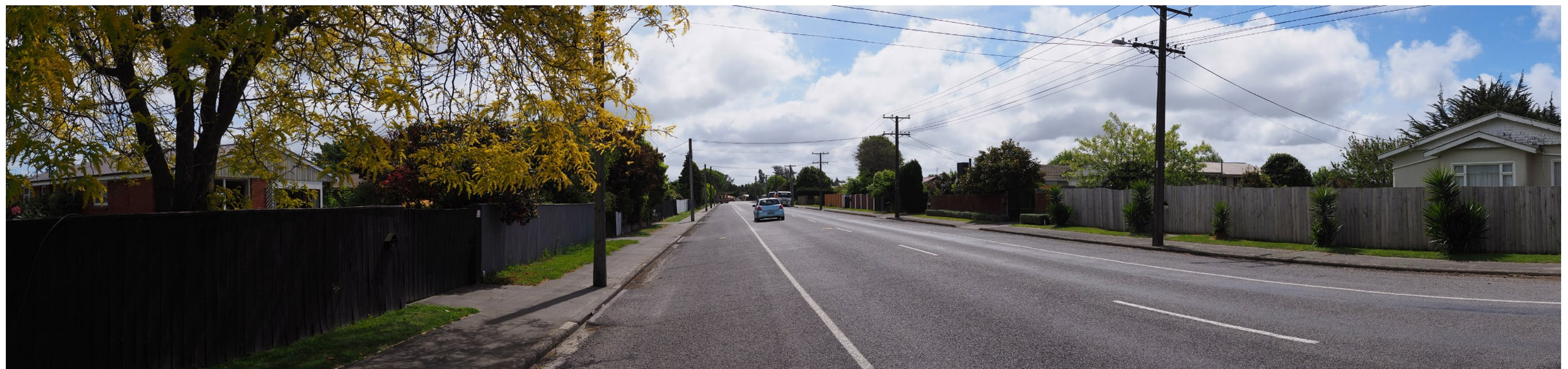
Viewpoint 11: Located beside 32 Marshs Road, looking west along the road alignment. The residential properties on the right hand side (north) will be zoned Heavy Industrial, which will allow for industrial development to replace these dwellings, which is 18m away.
