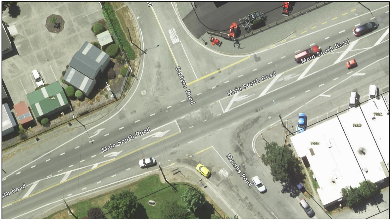
Figure 3-5. Aerial View of Layout of Main South Road / Marshs Road / Barters Road Intersection
