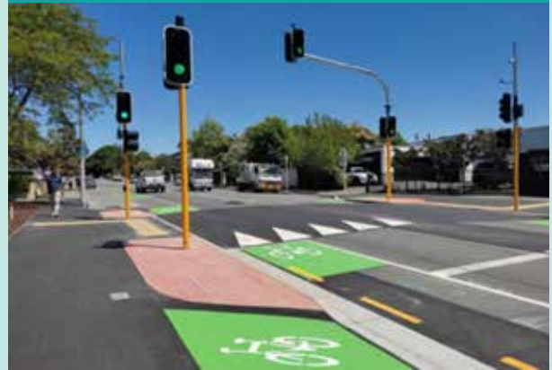
A pedestrian crossing on a safe speed platform, outside He Tiwai Mātauranga Heaton Normal Intermediate School on Heaton Street
