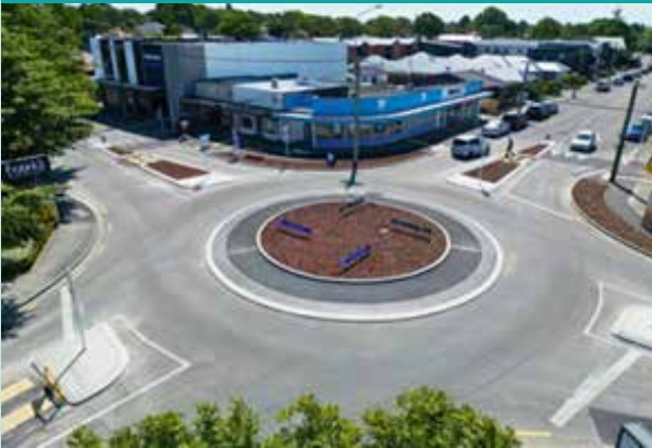
The Clyde Road / Ilam Road roundabout
