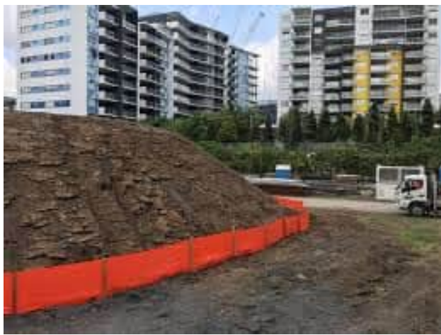
A silt fence around the base of a soil stockpile.
