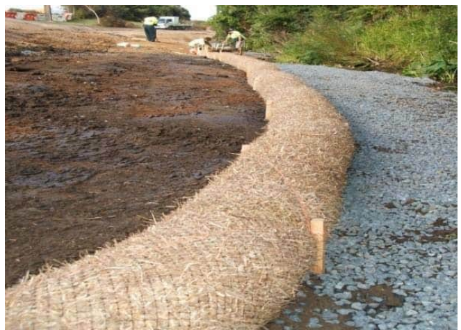
A hay bund around a stockpile.
