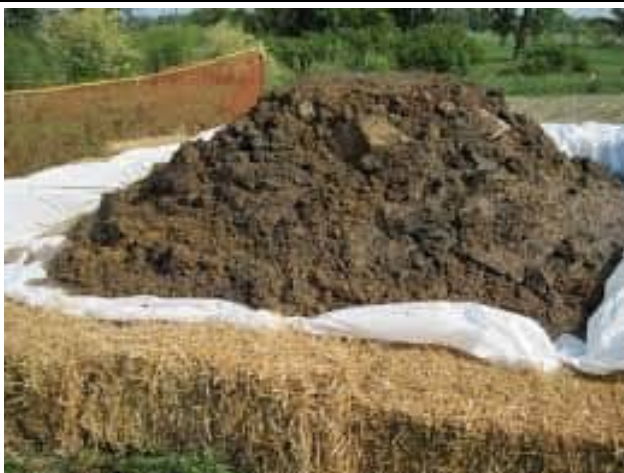
Haybales and a geotextile liner around a soil stockpile.
