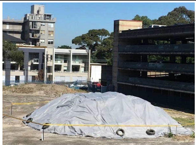
An impermeable cover on a stockpile.
