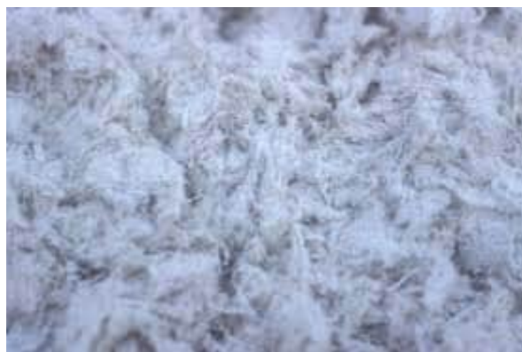
Loose fill asbestos insulation
