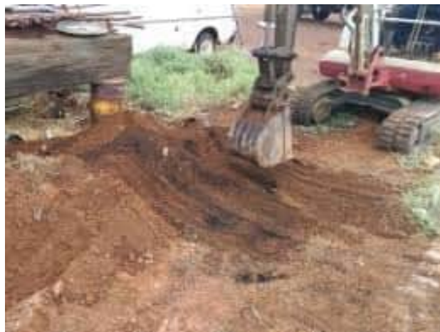
Areas of dark staining and unnatural colouration in a shallow excavation.
