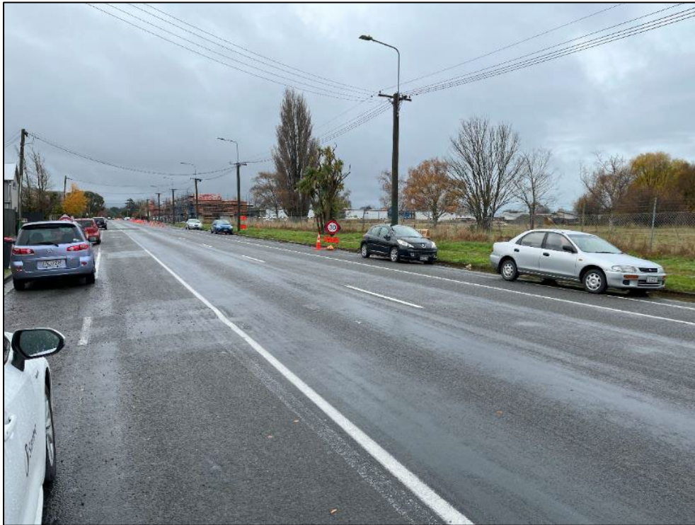
Photograph 3-1: Madras Street view North
