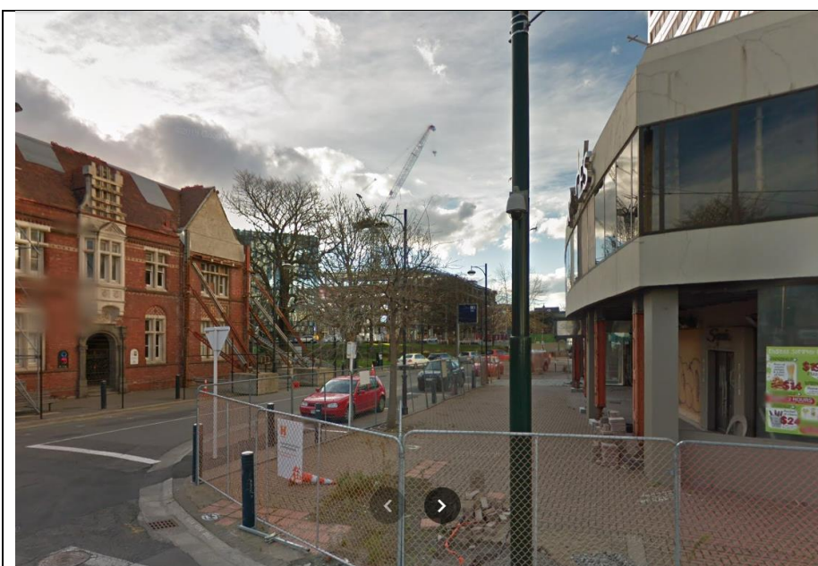
The ex-Rydges Hotel has a podium which greatly moderates its height at the street edge.
