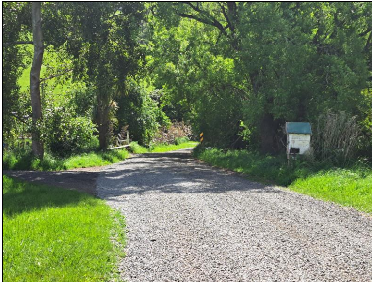
Figure 5: Wharf Road condition, unsealed.
