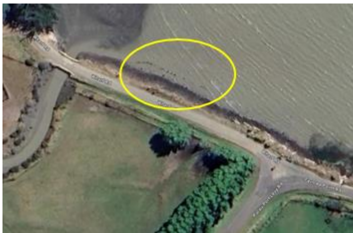
Figure 1: Aerial view of posts erected in the water and vegetation (reeds) planted as part of mitigation measures
