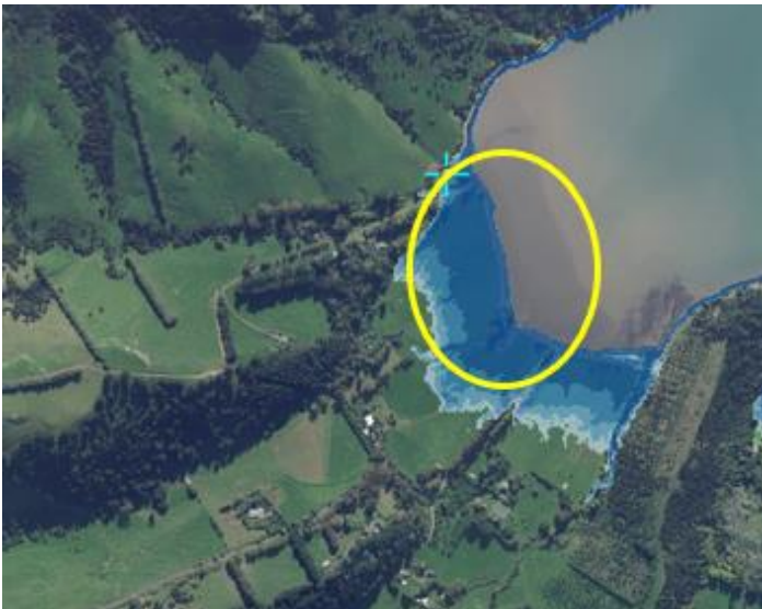
Figure 4: Section of Wharf Road affected by coastal flooding (approximately 500 metres).
