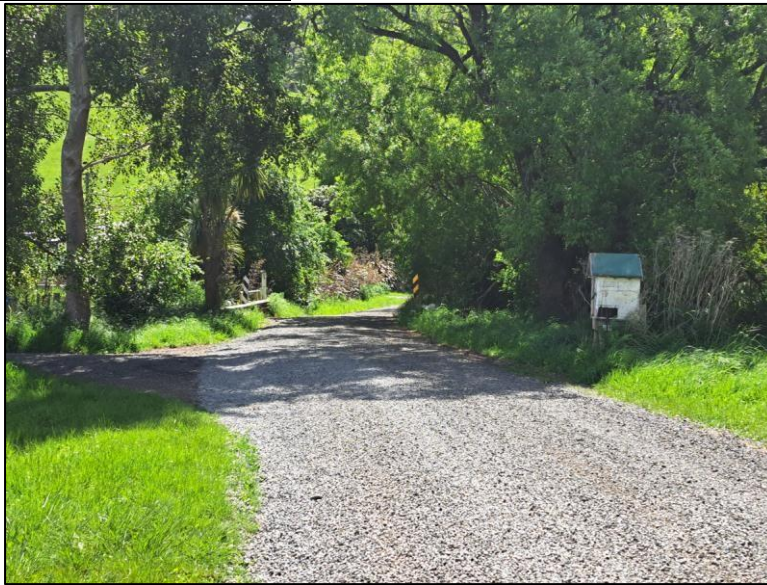
Figure 5: Wharf Road condition, unsealed.
