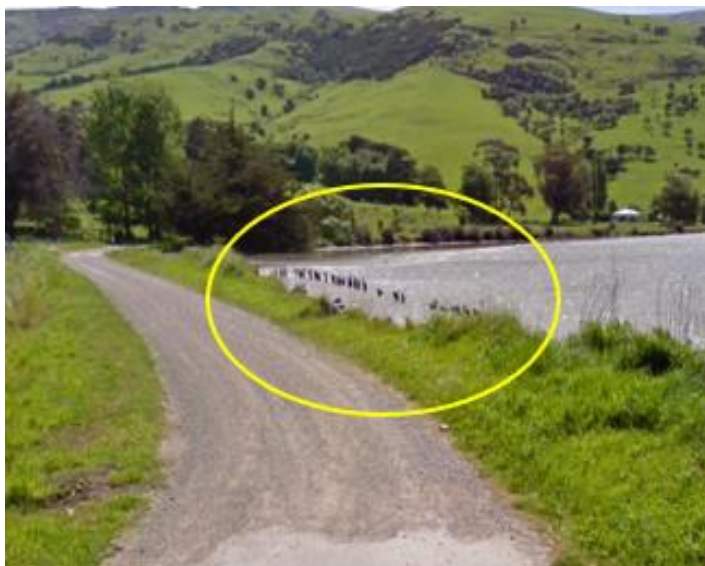
Figure 1A: Posts erected and vegetation (reeds) planted as part of mitigation measures
