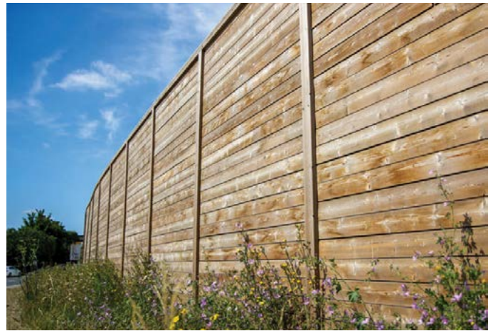
Precedent Images: Timber Acoustic Fence - Horizontal Palings
