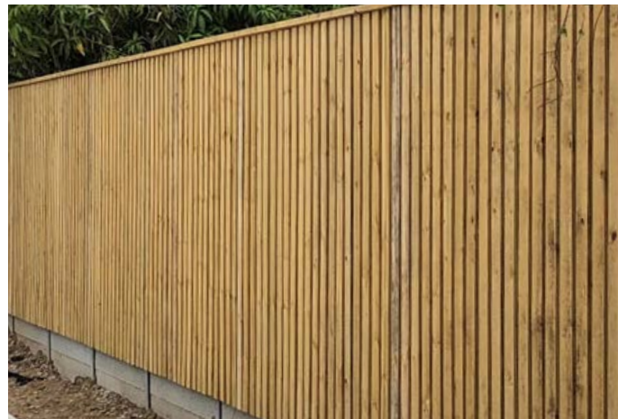
Precedent Images: Lapped and Capped Timber Paling Fence
