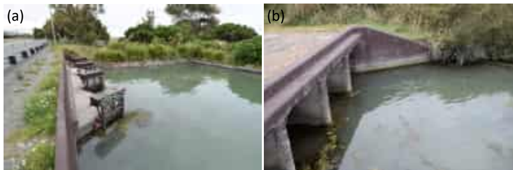
Figure 7. Linwood Canal outlet structure at the Avon Heathcote Estuary Ihutai on Humphrey's Drive. (a) View of the four flap-gates in operation on a high tide. (b) Tidal ingress into Linwood Canal through the southern culvert on an incoming tide.
