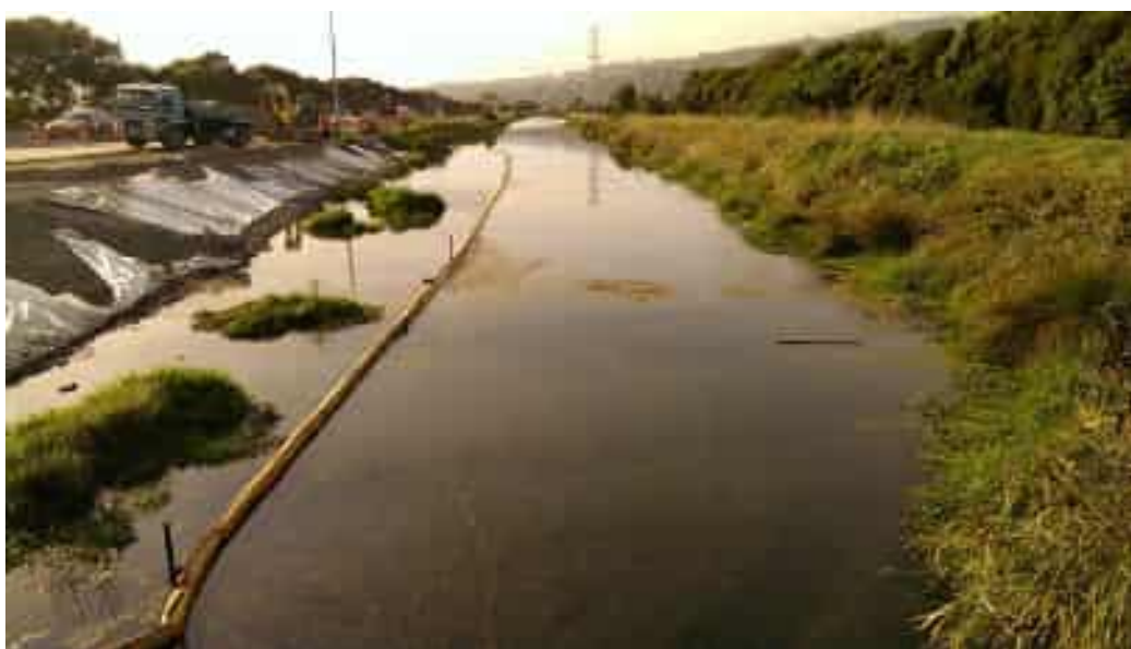
Figure 2. Linwood Canal looking downstream from Dyers Road showing current road works in the riparian zone. A silt curtain can be seen protecting the waterway from construction site run-off.
